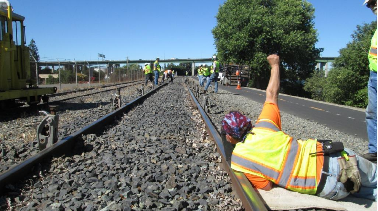
Joe looking through the sight-hole of the “hound” signals to Taka to stop cranking up the jack
