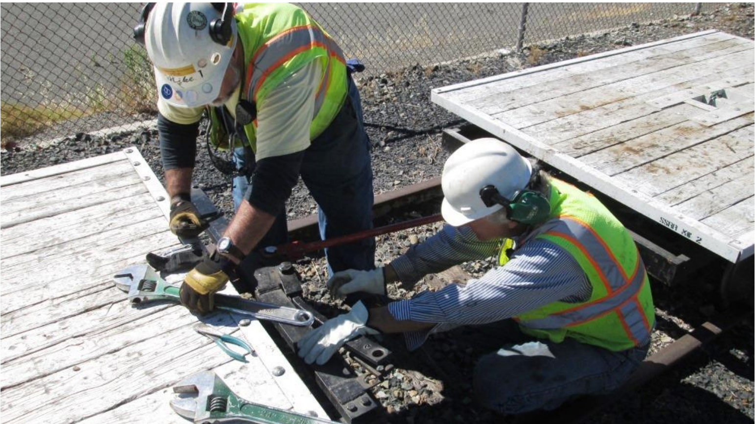
Meanwhile, Mike F. and Steve repair the bent draw-bar between the flatcars
