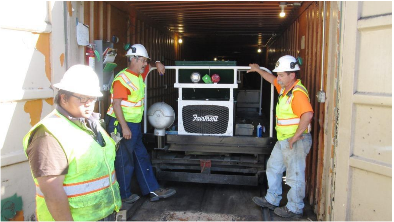
Ed and Joe discuss options for the repair of the motorcar while Anthony stands guard
