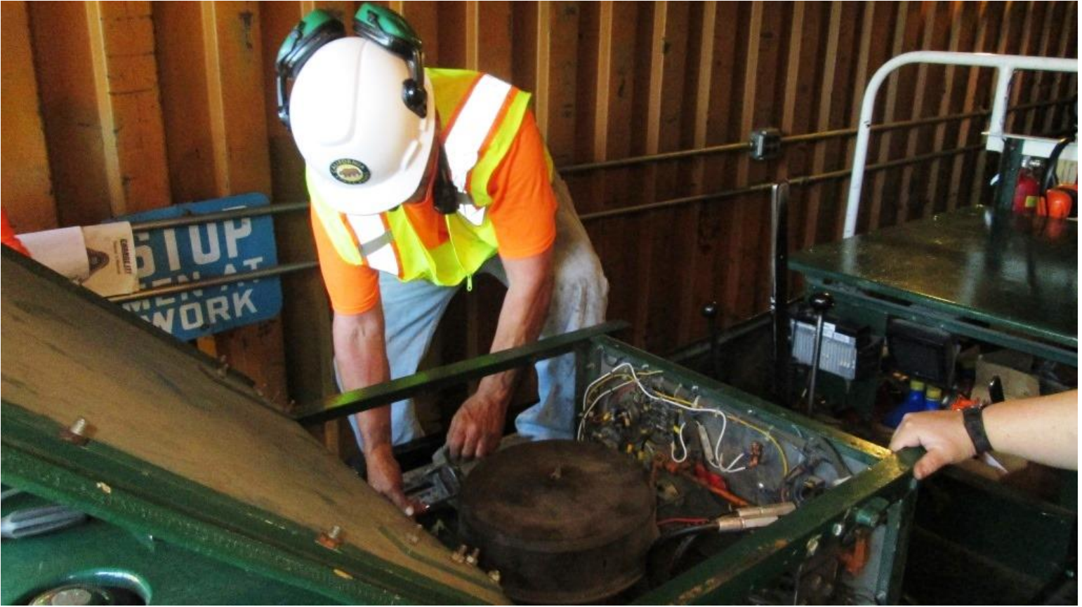
Joe finishes up installation of the ignition-coil on the motorcar
