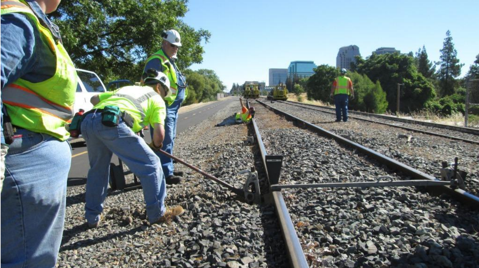
Taka cranks on the track-jack as Joe gives direction while sighting the level through the "hound"
