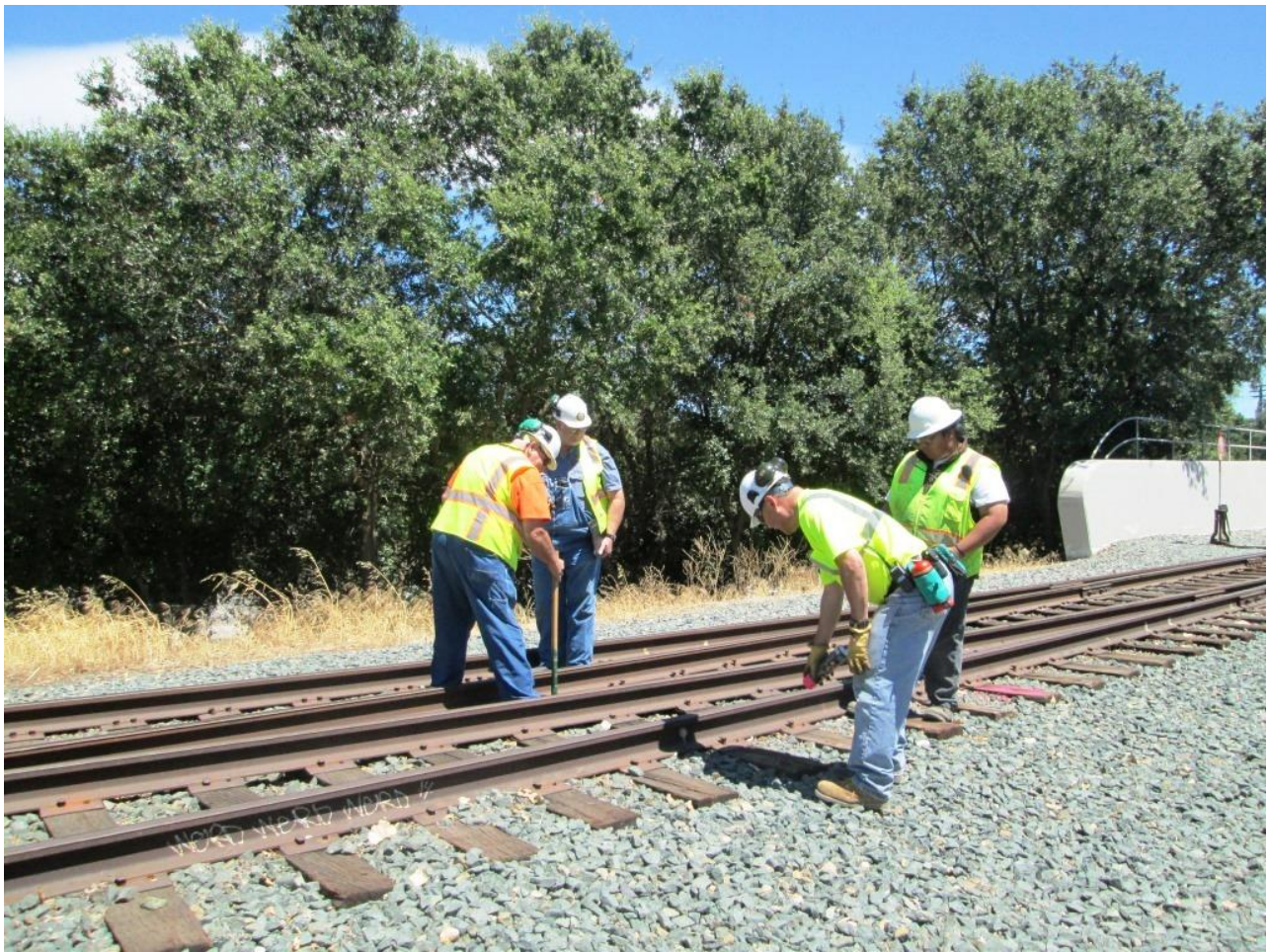
Harry taps a switch tie to test its solidity. Taka marks the bad ones with marker paint
