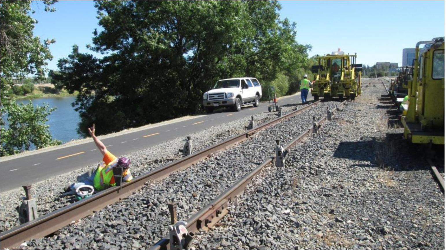
Frank starts tamping the track while Joe continues sighting the level with the “hound”
