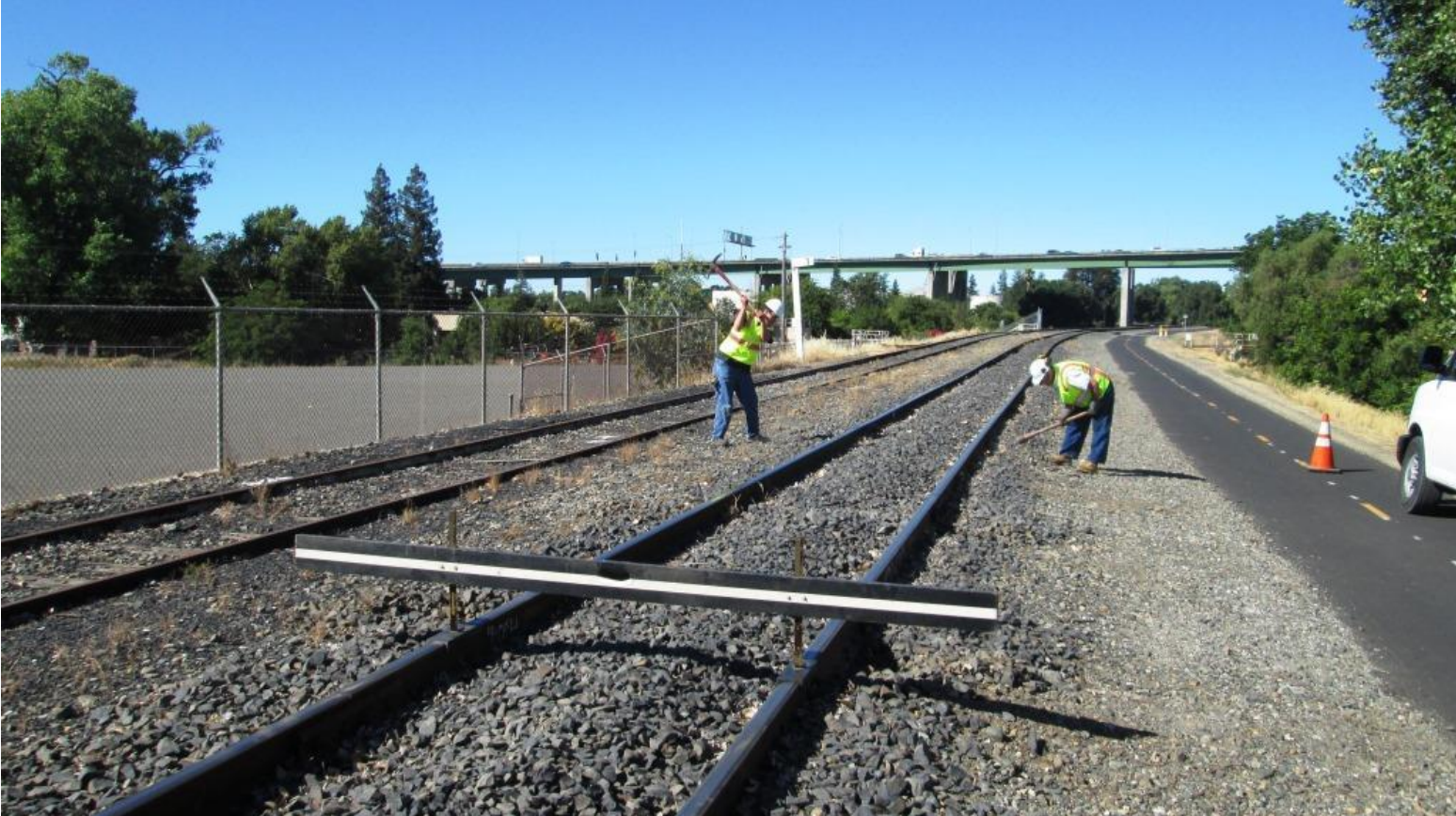
Weston and Clem dig out pockets for the track-jacks to be placed
