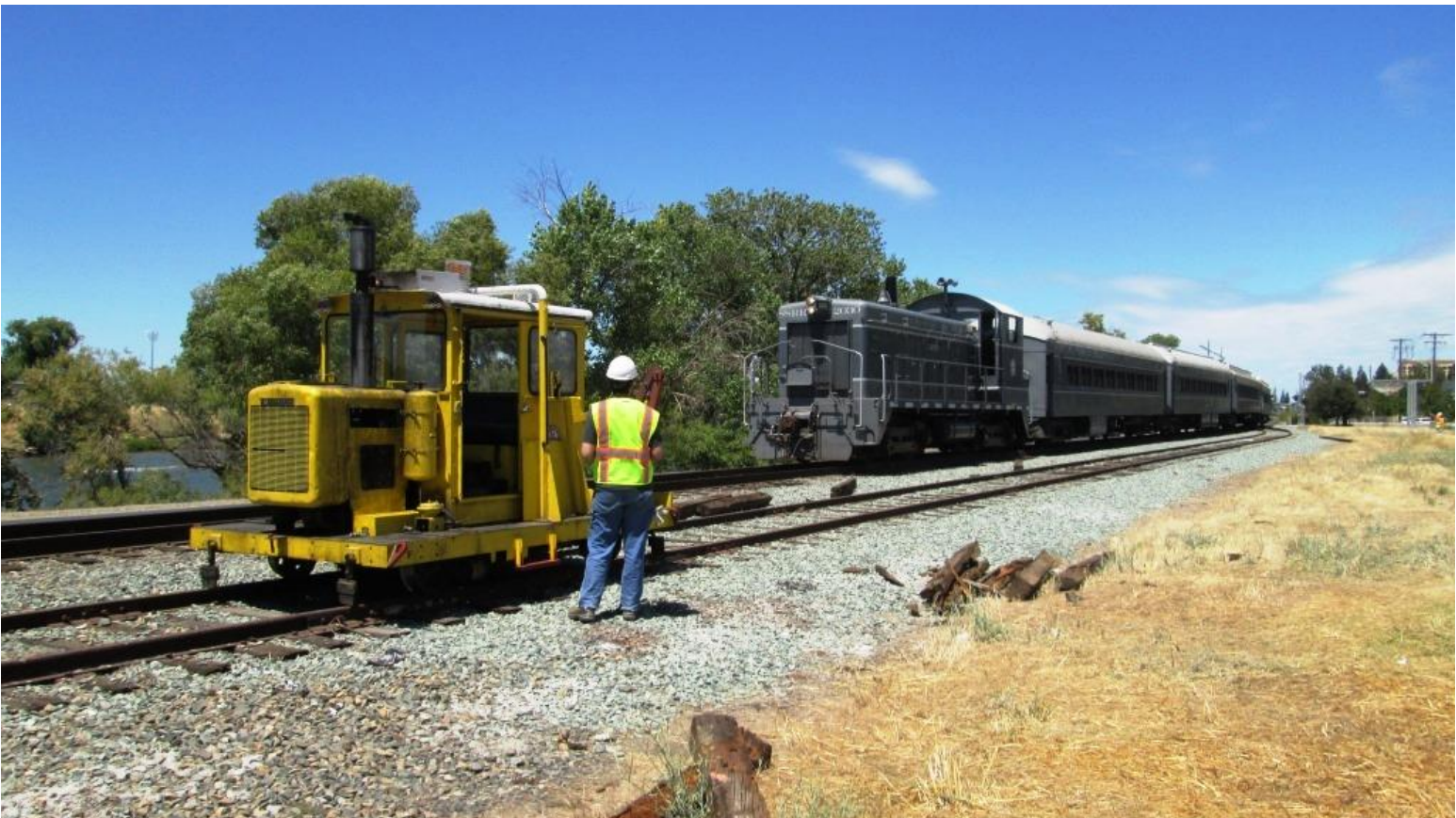
Weston watches the train pass by as the Team clears away dead ties
