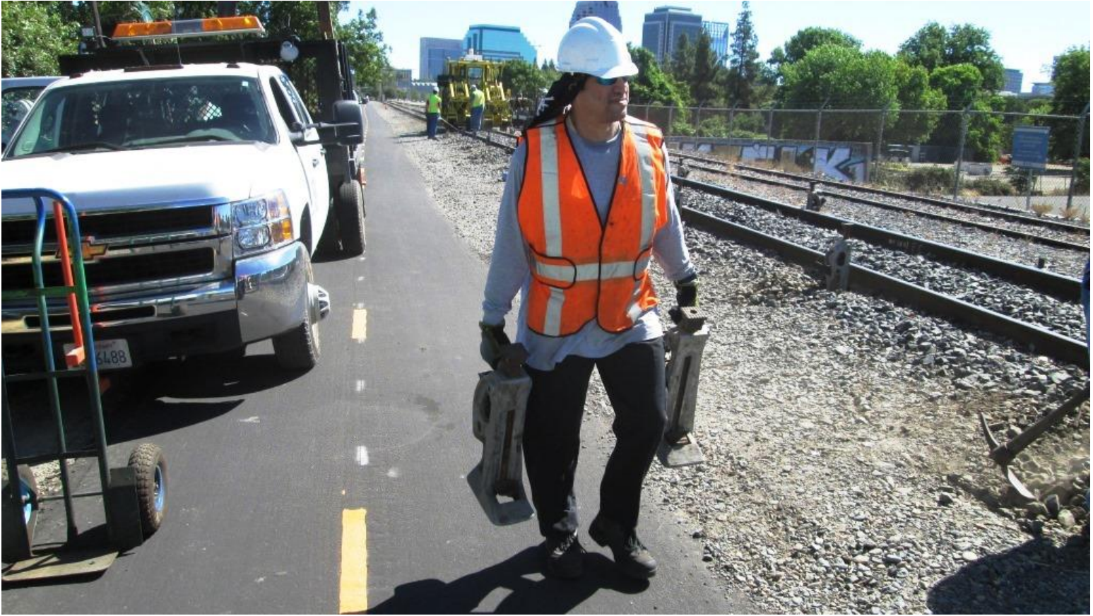
Jose then takes the jacks further down the line to reset as the leveling continues
